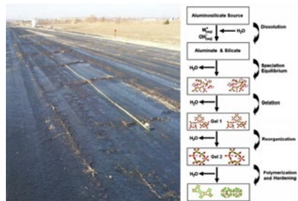
(left) Vertical heaves generated during the construction of U.S. 67 near Midlothian, Texas and (right) conceptual model of geopolymerization.
