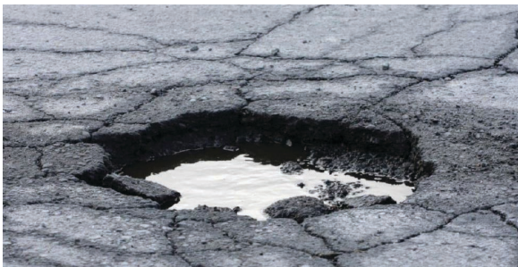
AC Stripping Damage in Flexible Pavement in Louisiana
