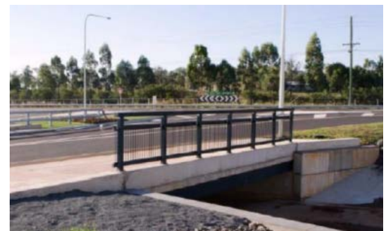
Figure 1. Bridges and pavements build using GPC concrete at Brisbane West Camp Airport, Australia
