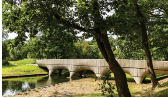
Figure 1. A 95-ft 3D printed concrete bridge in Nijmegen, Netherlands
