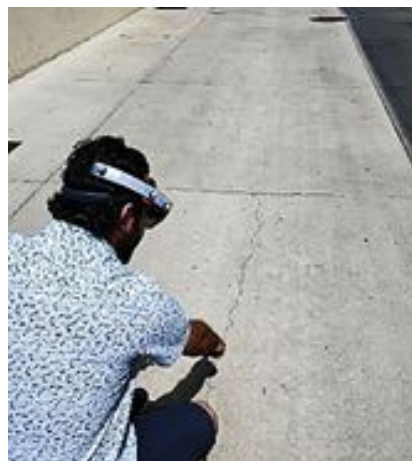
Inspector with AG headset analyzing crack on pavement.
