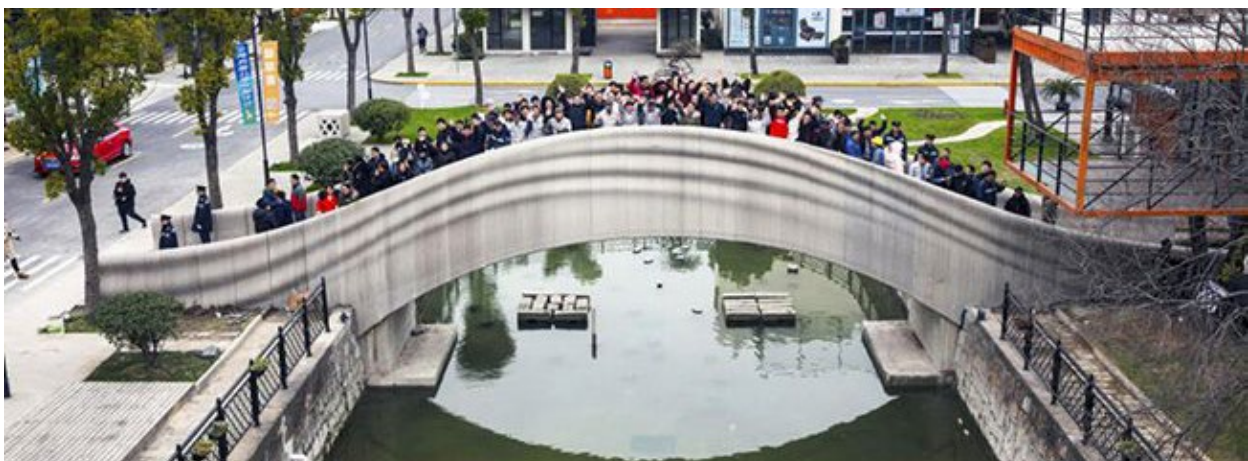
3D-printed bridge in China.
