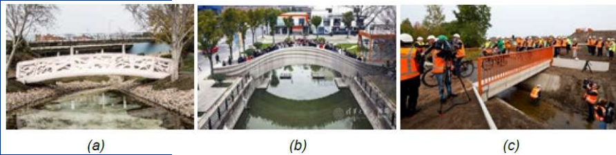
Figure 1. (a) 3D printed pedestrian bridge in Spain; (b) 3D printed bridge in China; and (c) 3D printed bridge in Netherland
