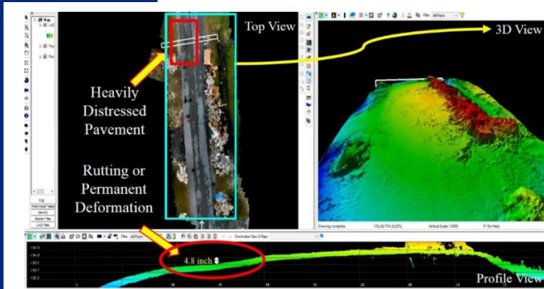
Figure 1. Photogrammetry Data Identifying Disaster Debris Volumes and Failure of a Pavement Section Immediately after Hurricane Harvey
