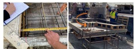
Figure 1. Rebar data Collection. Left: Measurement using tape (conventional); Right: Measurement by LIDAR scanner (proposed automation).
