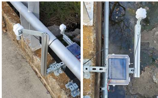
Figure 3. Installed UWLD systems on the pavement side and streamside
