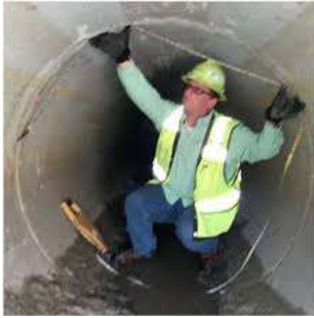
Figure 1: RC Sewer pipeline being inspected
