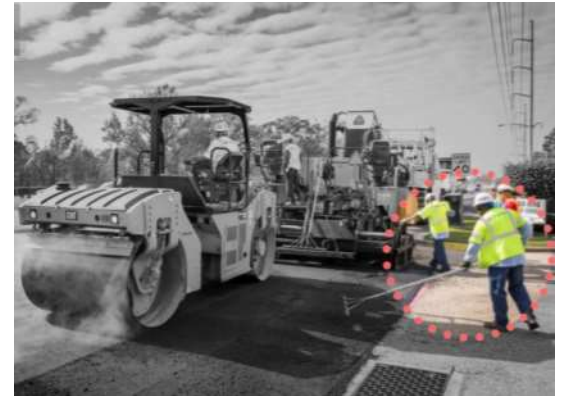
Figure 1: Road construction workers, exposed to multiple struck-by hazards
