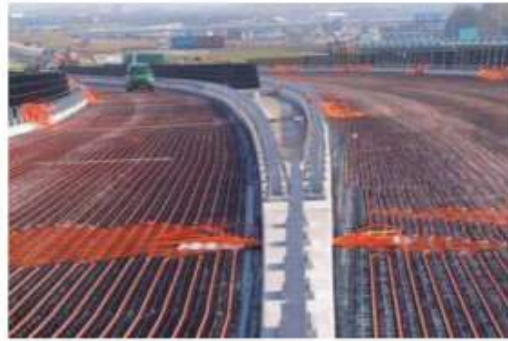
Figure 1: Asphalt Solar Collector System (De Bondt 2003)
