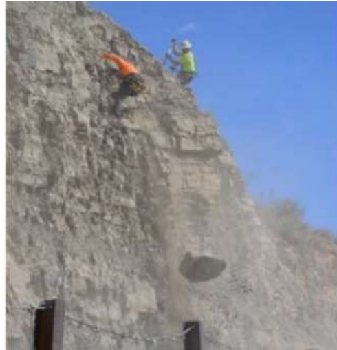
Figure 1: Rock fall mitigation Otero County, New Mexico
