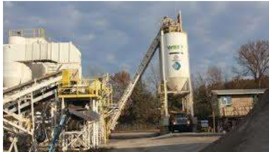
Figure 1: A Reclaimed Asphalt Pavement mix being developed at a plant.
