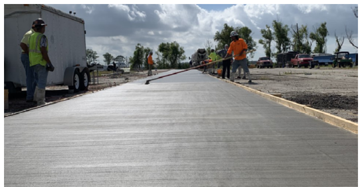
Construction of the ECC overlay
