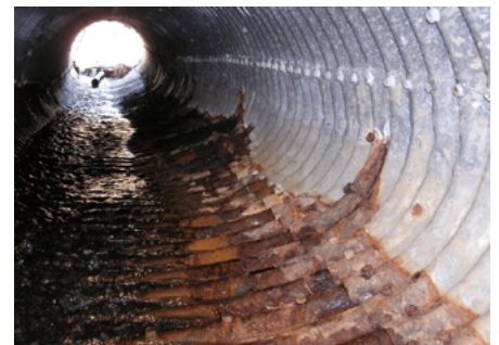
Corrosion of corrugated metal culvert
