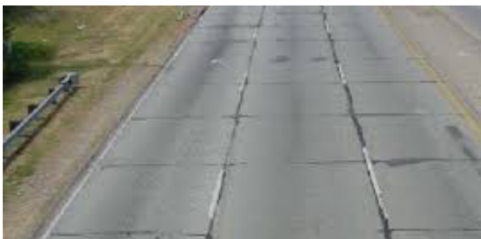
Example of reflective cracking
