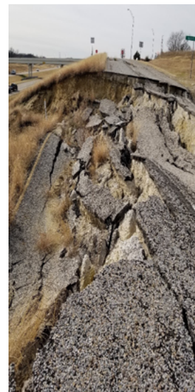
Embankment failure in Texas (site included in study)
