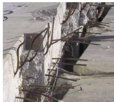
Damage to bridge supports during Hurricane Katrina
