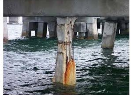
Figure 1. Reinforced concrete bridge affected by salt-water corrosion.
