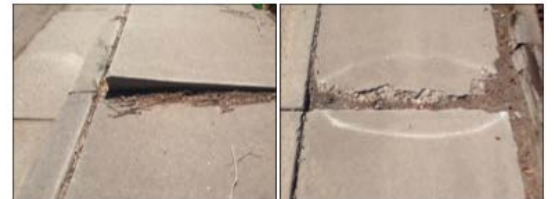
Figure 1. Typical sidewalk defects in Albuquerque.
