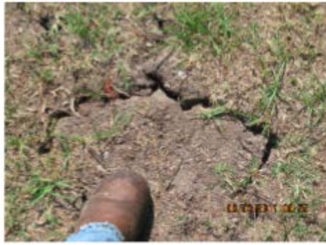
Figure 2. Photo of desiccation cracks along Louisiana Highway 327.
