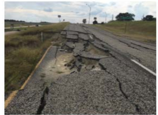
Figure 1. Slope failure in Grayson County, Texas.
