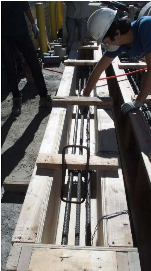
Figure 2. Student placing reinforcement into formwork.
