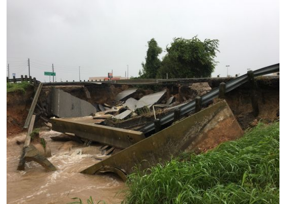
Figure 1. Bridge collapse near Rosenberg, TX as a result of Hurricane Harvey (Photo: Rick Jervis, USA TODAY 2017).
