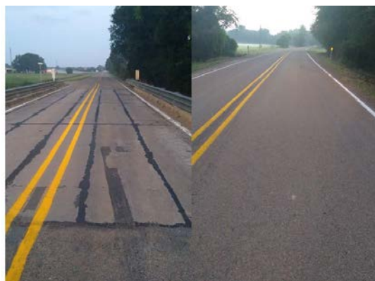
Figure 2. Field section before and after chip seal application.
