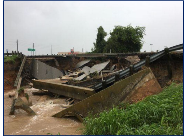
Bridge collapse as a result of Hurricane Harvey
