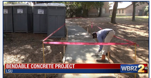
Sidewalk installation utilizing ECC as on the local news
