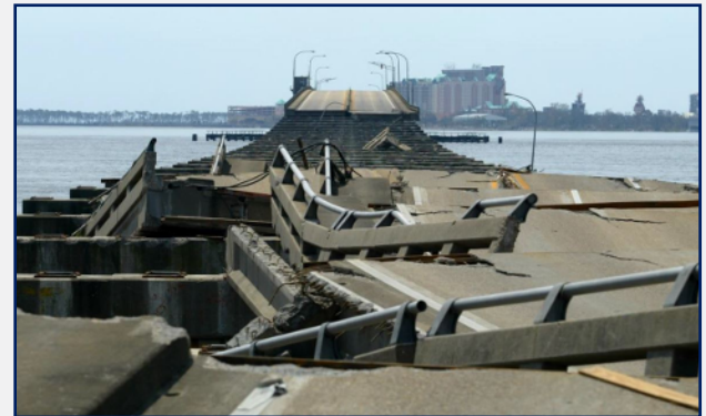
Damage to bridge caused by Hurricane Katrina
