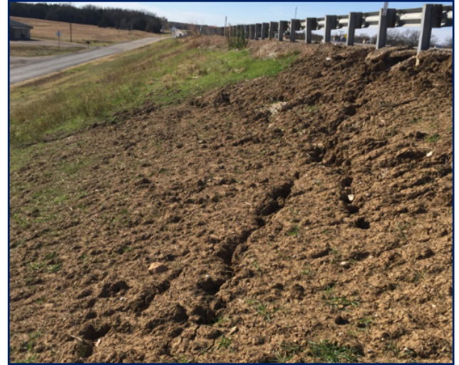
Tension cracks along embankment slope at Texas site
