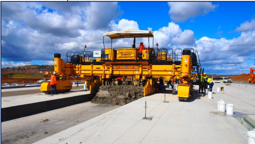
Geopolymer concrete being place
