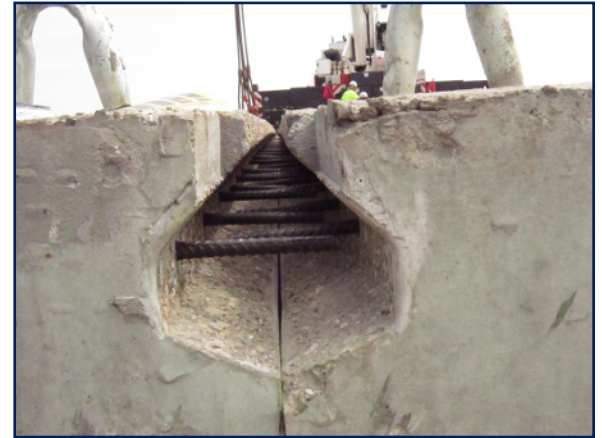
Example of bridge shear keys with dowels
