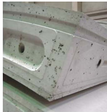
Traditional Concrete CVC
