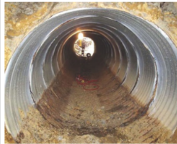
Corroded Metal Culvert Cross-Section
