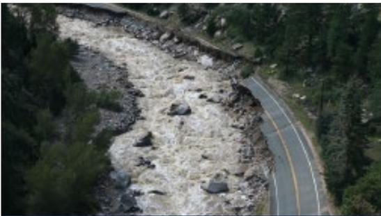
In September 2013, flood damage on US-34 destroyed an entire section of roadway.
